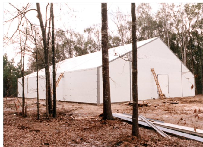
Compaq Computer chose a foam core panel building to assure RFI/EMI compliance for attenuation.
