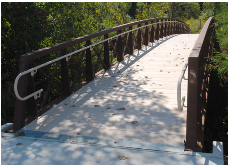
Above: A bridge that connects the Frog Hollow Nature Trail with adjoining trails and recreation areas in Jefferson City, Missouri is refurbished using STRONGDEK™ to replace structurally-deficient steel bridge decking.
