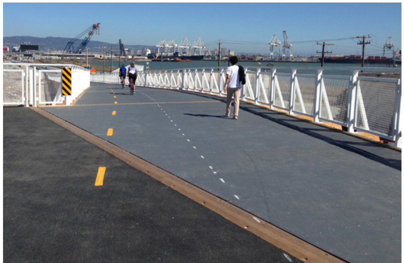
Left / Above: The San Francisco-Oakland Bay Bridge and Biking path in California utilized EXTREN® 1/8" thick plate for its walking/biking surface.
