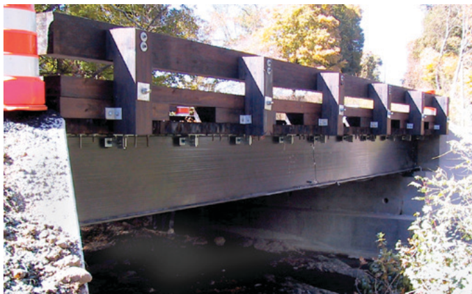
Above: The 36" x 18" EXTREN DWB® was installed in a Federal Highway Administration (FHWA) sponsored demonstration bridge project as part of the Innovative Bridge Research and Construction Program (IBRC) in September 2001. University professors from Virginia Tech performed a series of tests on the 36" x 18" EXTREN DWB® including stiffness testing of each beam. Eight beams were selected for the 38' span AASHTO HS-20 bridge located on Route 601 in Sugar Grove, Virginia.
