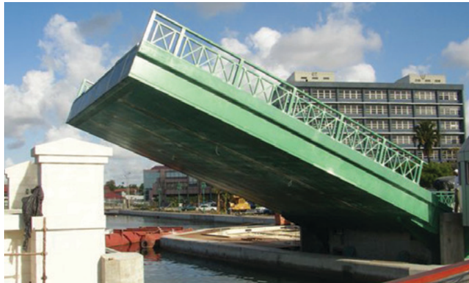
Above Left / Left: An all-composite bascule bridge in Bridgetown, Barbados, was built using Strongwell's COMPOSOLITE®, COMPOSOLITE HD™, and EXTREN® structural shapes. The drawbridge is mainly used by pedestrians in this tourist destination.
