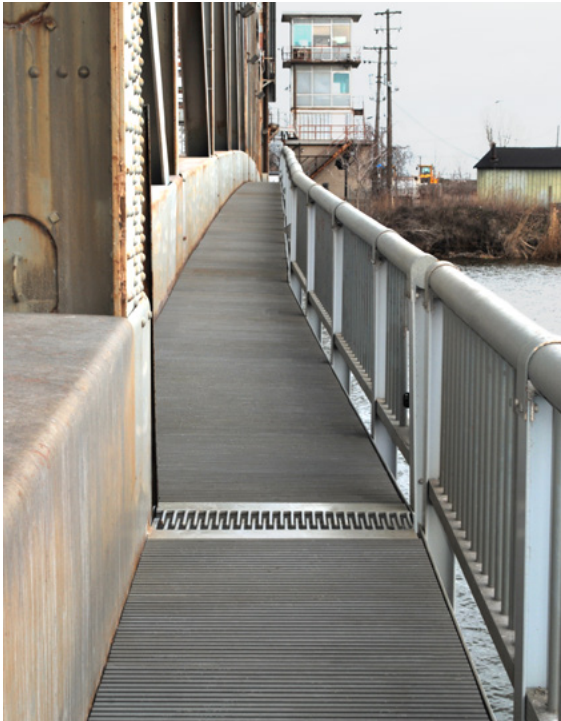
Left / Below: The Cleveland Lift Bridge in Cleveland, Ohio utilized DURADEK® T-5000 pultruded grating to replace metal pedestrian walking surface which had rusted away.
