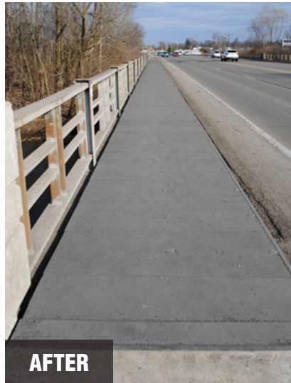
Above: A walkway on Refugee Road over Beaver Creek in Franklin County, Ohio, uses SAFPLANK® along with EXTREN® structural supports.
