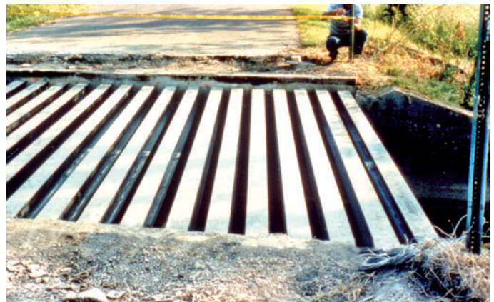
Above: Tom's Creek Bridge, Blacksburg, Virginia, reopened to traffic June 23, 1997 as one of the first composite short-span vehicular bridges in the U.S. After replacing the corroded steel beams supporting the bridge with 8" x 6" composite beams, the 17-1/2 ft. x 22 ft.-wide bridge was upgraded from 10-ton capacity to 20-ton capacity. More than 1,000 cars per day cross the bridge.
